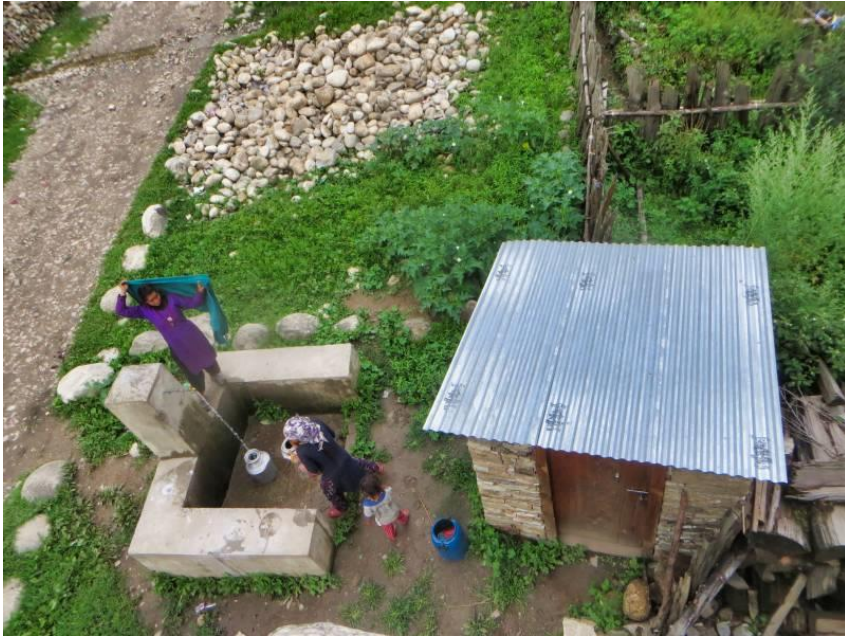
Pic.13. Pere families using a DWS tap stand constructed as part of the GG1.
