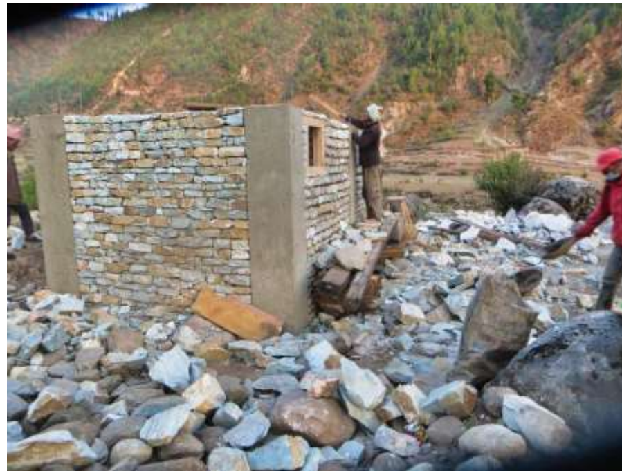
PIC.54. Solar Hot Water Bathing Center under construction.
