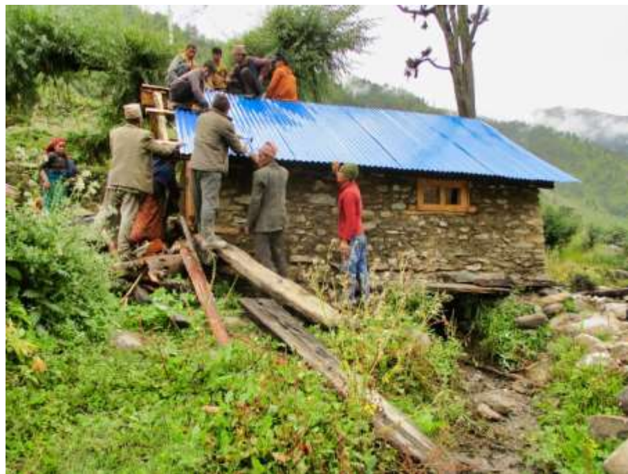
PIC.47. A newly constructed IWM stone and mud house.
