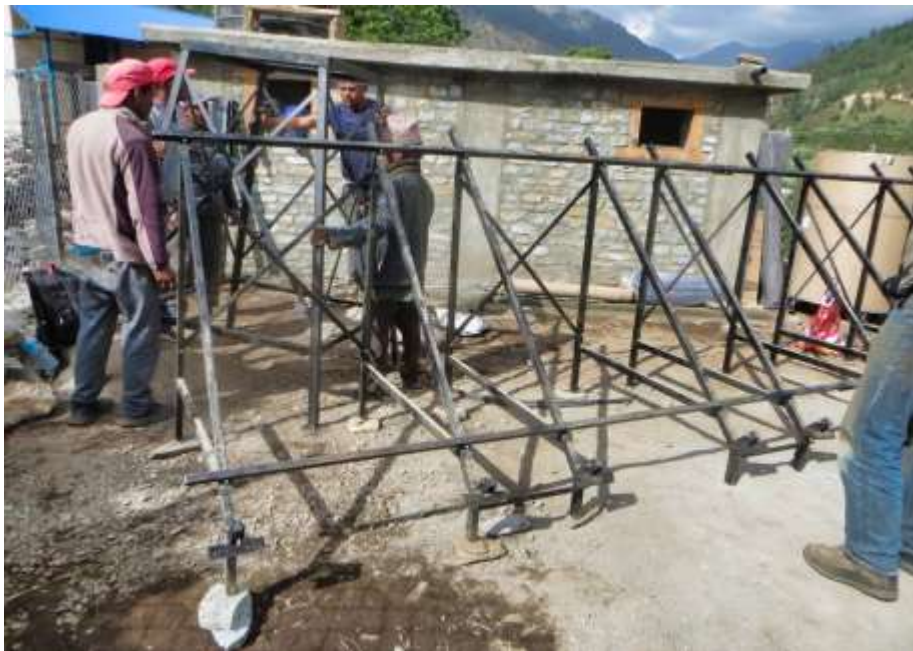
PIC.57. Solar Hot Water Bathing Center under construction.
