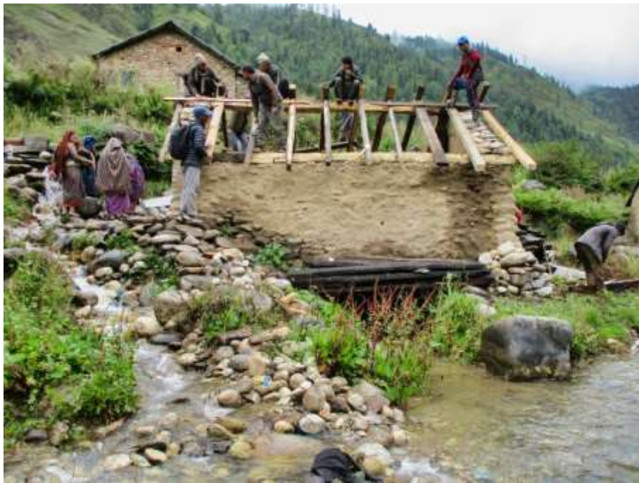
PIC.45. The improved Water Mill's stone and mud house under construction.
