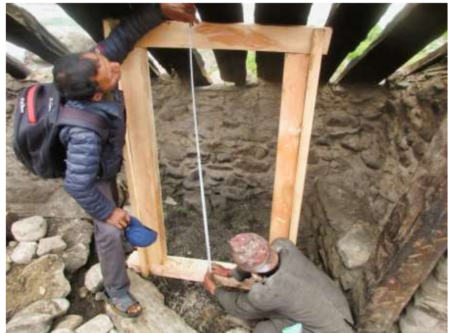
PIC.44. Improved Water Mill (IWM) house under construction.
