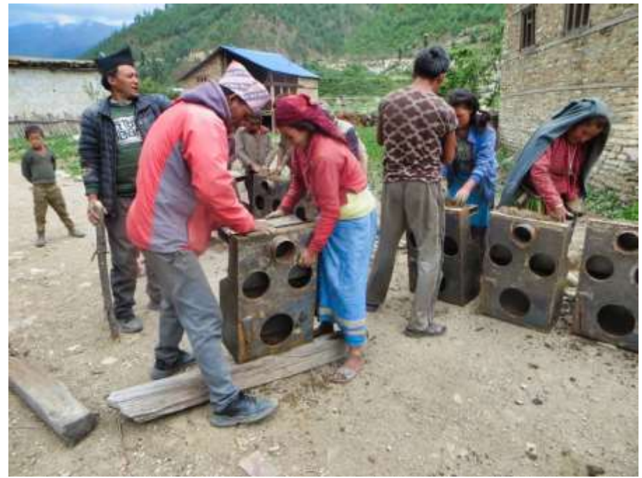
PIC.26. RIDS-Nepal staff is teaching the correct SMS installation process.
