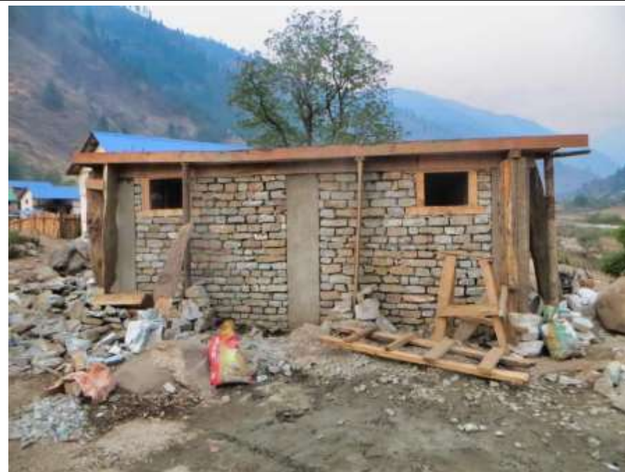
PIC.56. Solar Hot Water Bathing Center under constructions.
