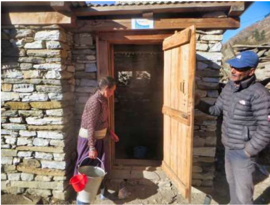
PIC.17. RIDS-Nepal Staff follow up a Pit latrine constructed as part of GG1.
