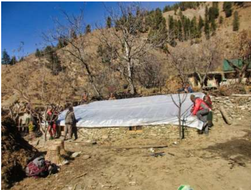
PIC.35. RIDS-Nepal teaching how to cover the GH with the UV stabilized plastic.
