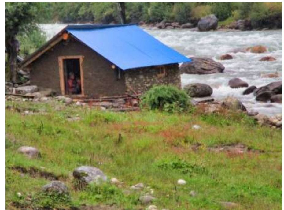
PIC.48. A newly constructed IWM stone and mud house.
