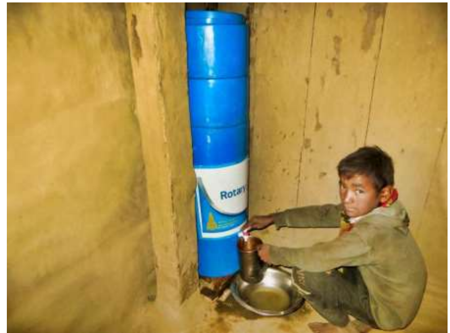
PIC.42. A boy using the new Slow Sand Water Filter (SSWF) after installation.
