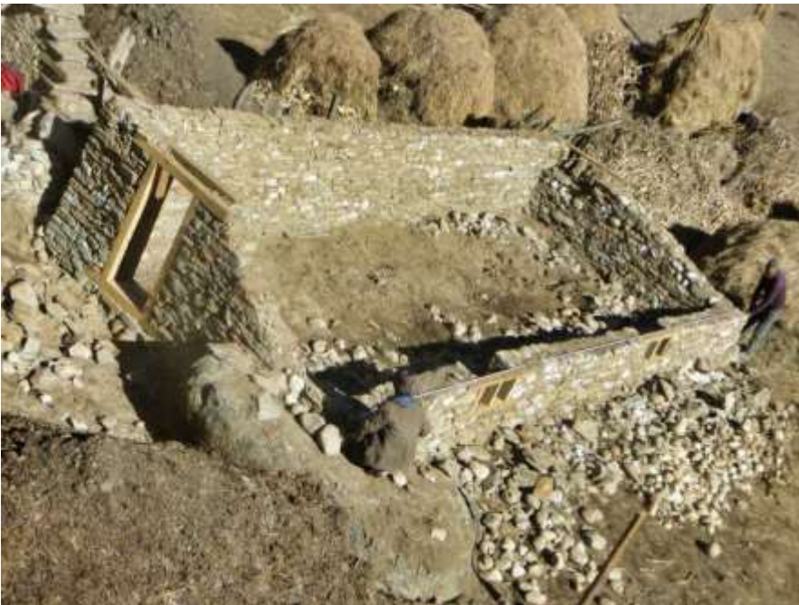
PIC.31. The foundation of a newly started Pere High-Altitude Green House.
